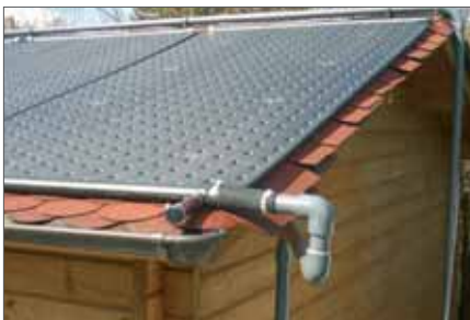
Sloping roof installation
