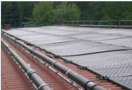
Flat roof installation
