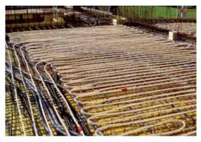
Roth Isocore concrete core temperature control
