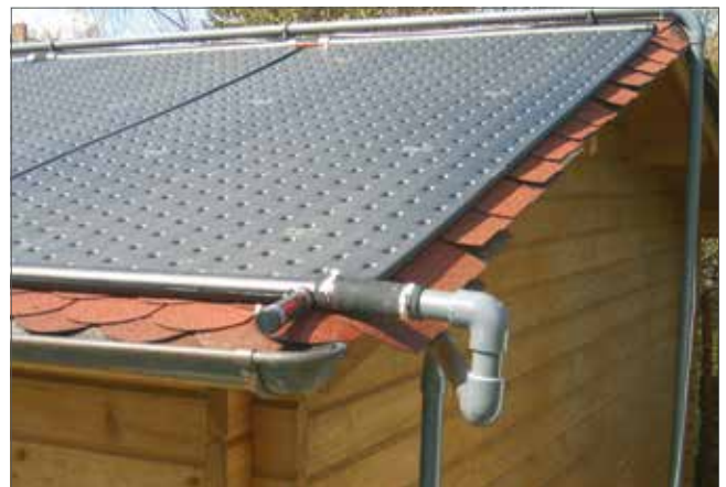
Sloping roof installation
