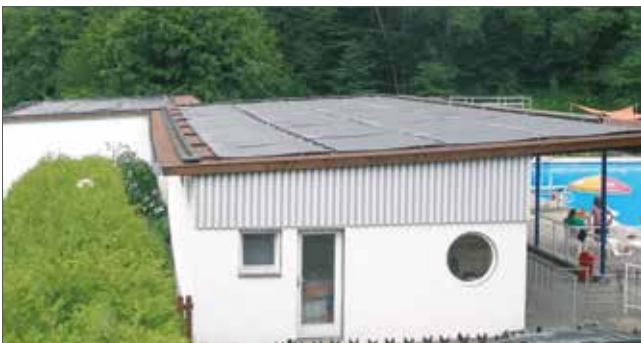
Roof installation at the Holzhausen swimming pool
