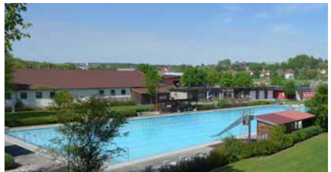
Roof installation at the Arnstorf swimming pool
