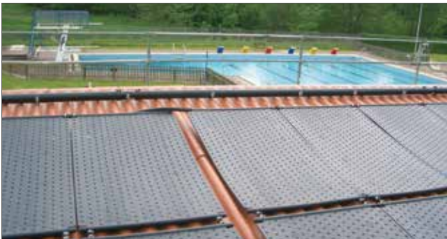
Roof installation at the Knüllwald-Remsfeld swimming pool
