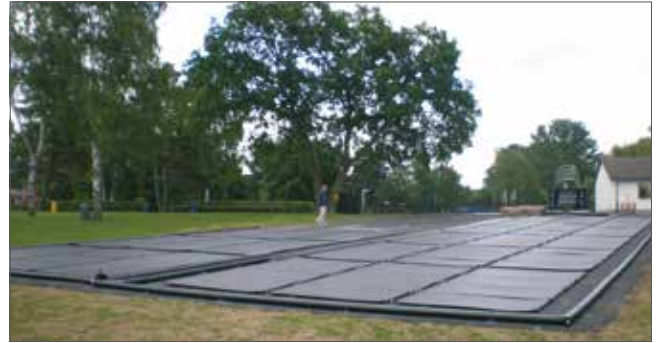
Open space installation at the Wehrheim swimming pool
