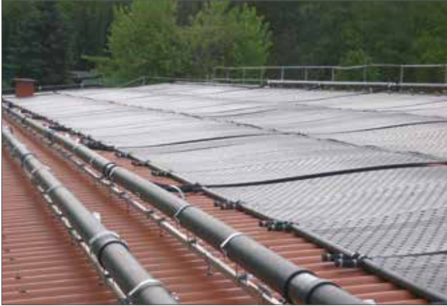
Flat roof installation
