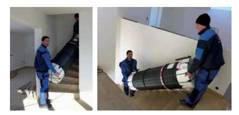
The plastic heat storage tank is just a third of the weight of a conventional steel storage tank, making it easier to transport up and down stairs.
