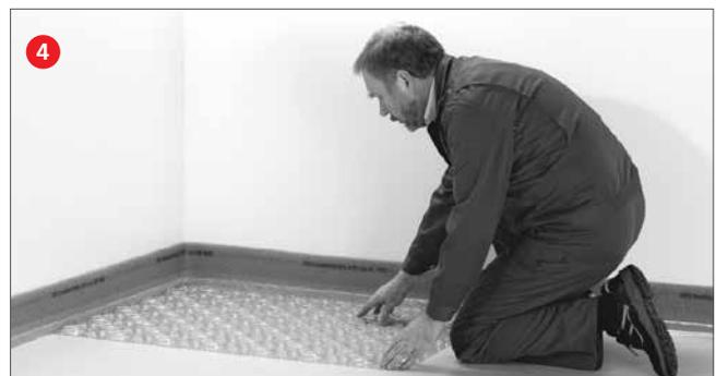
5. Roth KlimaComfort® Compact System panels have specially designed edges so the next panel can be laid adjacent to the previous one with a slight overlap.
