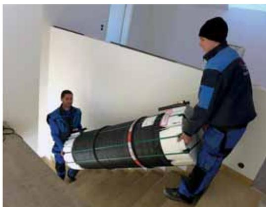
The plastic heat storage tank is just a third of the weight of a conventional steel storage tank, making it easier to transport up and down stairs.
