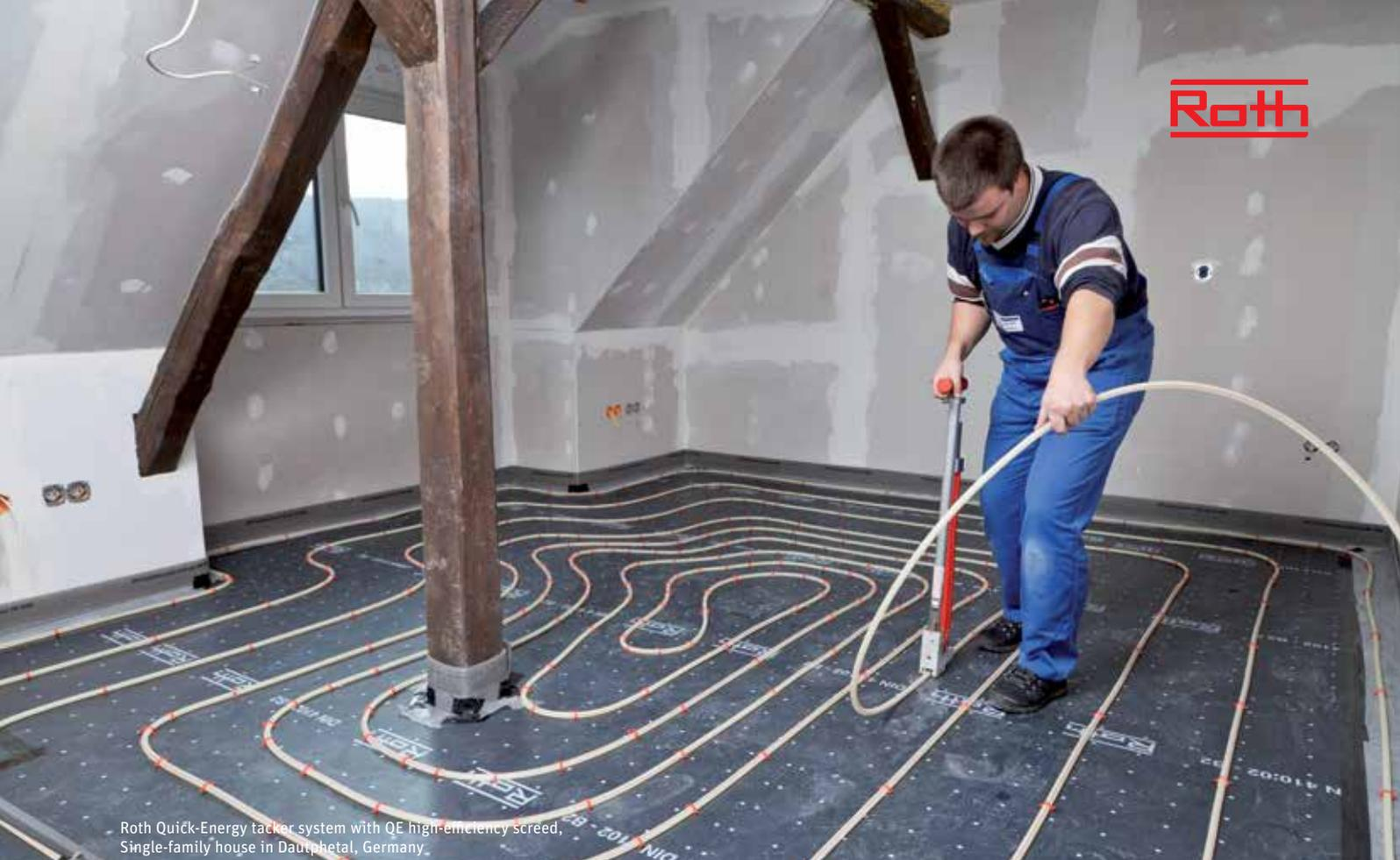
Roth Quick-Energy tacker system with QE high-efficiency screed, Single-family house in Dautphetal, Germany.
