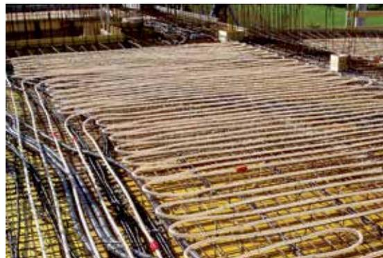
Roth Isocore concrete core temperature control
