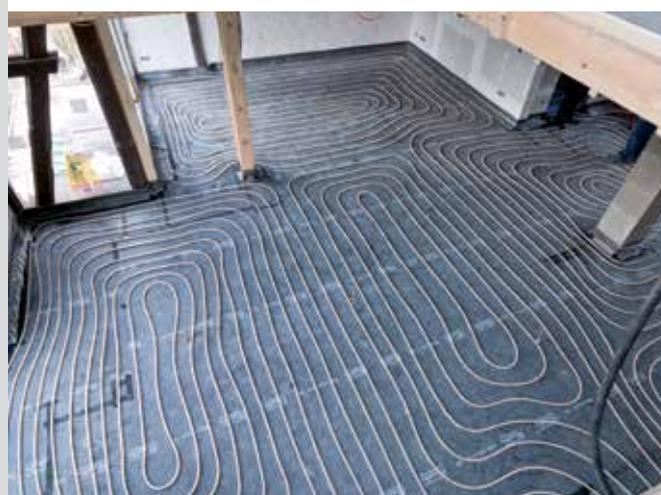
10 **Roth Isocore concrete core temperature control**
