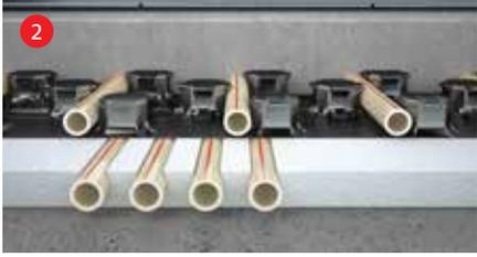
2 Floor construction without smoothing layer or additional insulation
