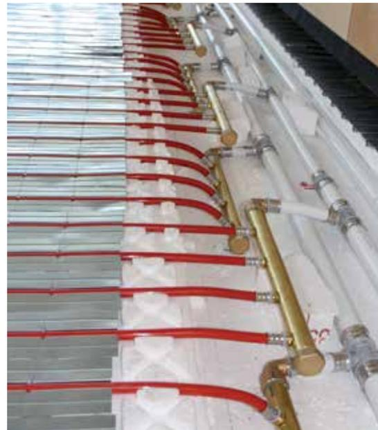
The heating circuit for the Roth ClimaComfort TBS radiant heating system in the Hinterlandhalle in Dautphetal is connected using a Tichelmann distribution network
